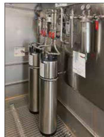
Fig. 2: MoHyPer integrated ultra-pure water system
